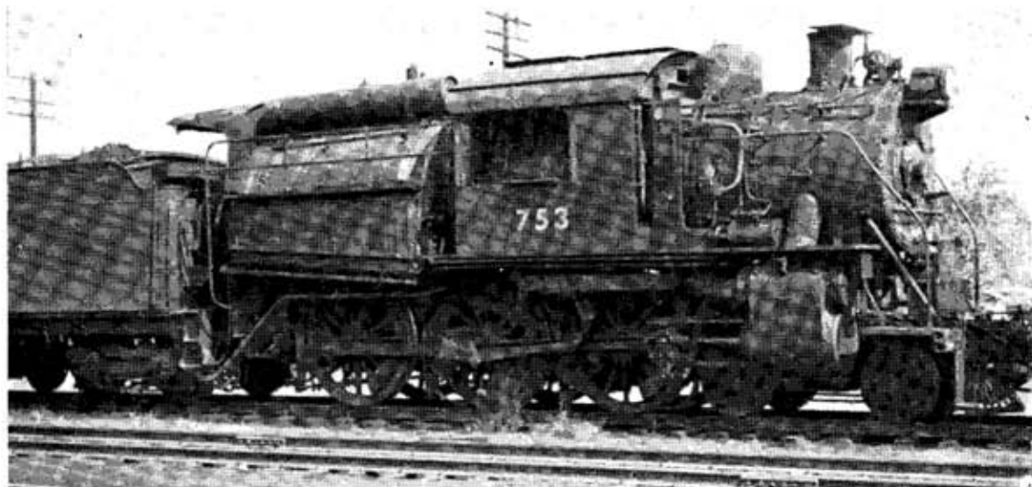
Fig. 3: Ten-wheeler No. 753 of the CRR OF N.J. waits for Monday morning commuter rush. Note that the engineer gained access to the cab from the front.
