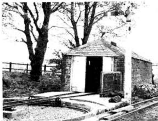
Below: The locomotive running shed which has two roads, and one of the signals.
