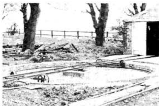
The turntable or transhipper which serves five roads, in its skeleton form.
