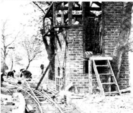
Below: The partly completed signal cabin and island platform.
