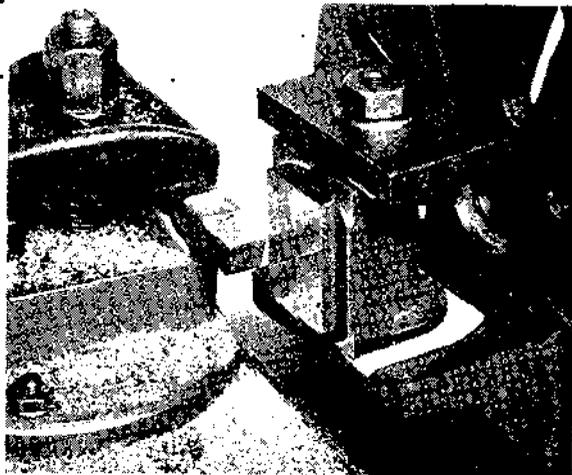
*Third operation. The cylinder is mounted on the angle plate for machining the valve face*
