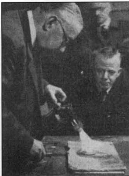
Melting the silver in depression ring.
