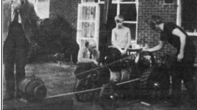
The Burrell doing some actual generating
