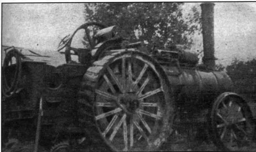
Fig 28. 8 n.h.p. traction engine by Harvey & Williams Ltd.
