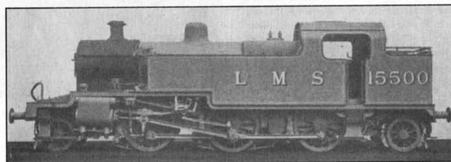
One of the New Series of L.M.S. 2-6-2 Tank Locos.
