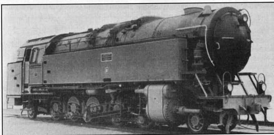
New 2-10-2 Tank Engine built by Borsig, of Berlin, weight 136 tons.
