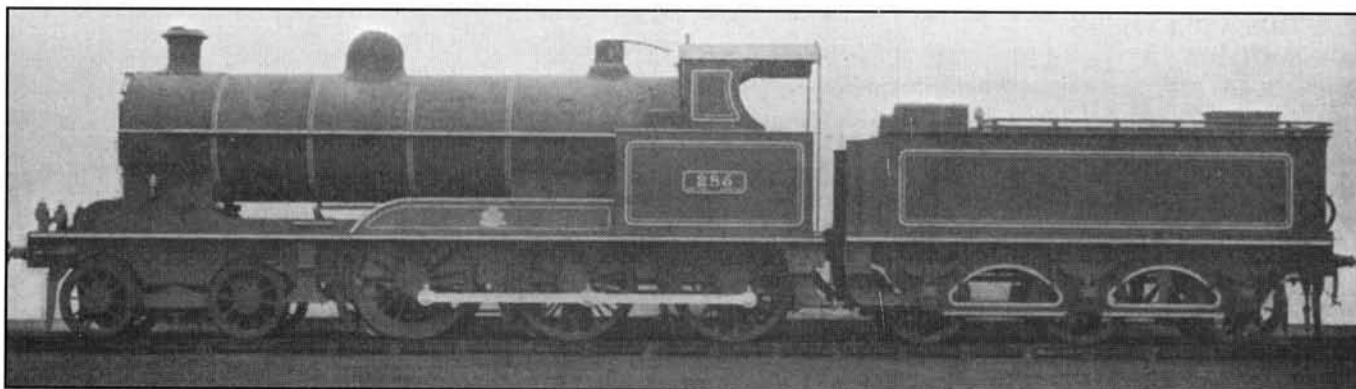
4-6-0 TYPE FAST GOODS LOCOMOTIVE: LONDON & NORTH-WESTERN RAILWAY.
