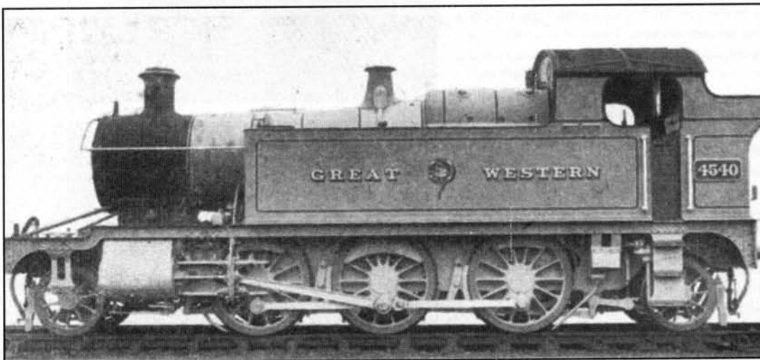
NEW 2-6-2 TYPE TANK ENGINE: GREAT WESTERN RAILWAY.
