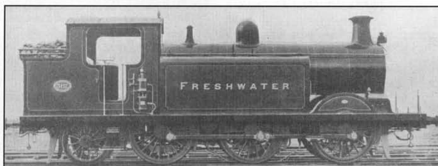
FIG.23—L.B. & S.C.R. SIX-COUPLED PASSENGER TANK LOCOMOTIVE.
