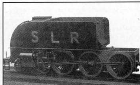
One of the driving units of the Garratt-style locomotive
