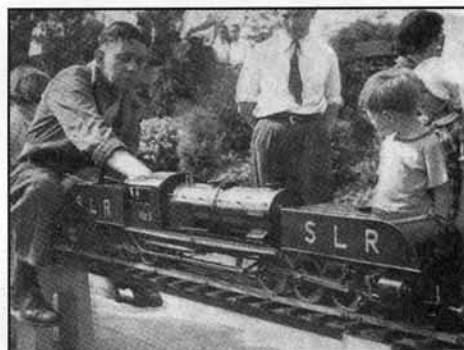
Gemini is seen here prepared for a run on the Watford club's track at Chipperfield. Note top-feed for the donkey pump – not yet fitted.
